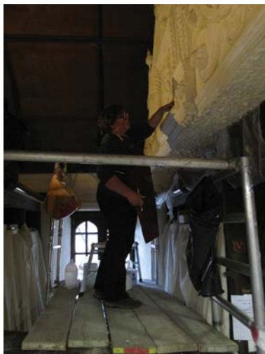
Cliveden Conservation restored the water-damaged plaster frieze
